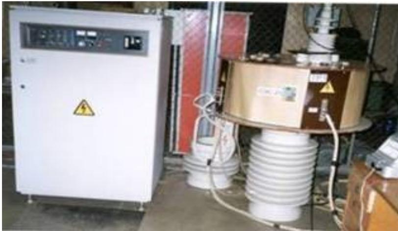
An industrial 25 kW frequency converter, which was used by us for designing the new device, had water cooling. It was inconvenient for autonomous use. In order to obtain a three-phase network of 50 Hertz at the outlet of the system, design of a P-22 frequency converter was changed and improved and three monophasic chokes for
